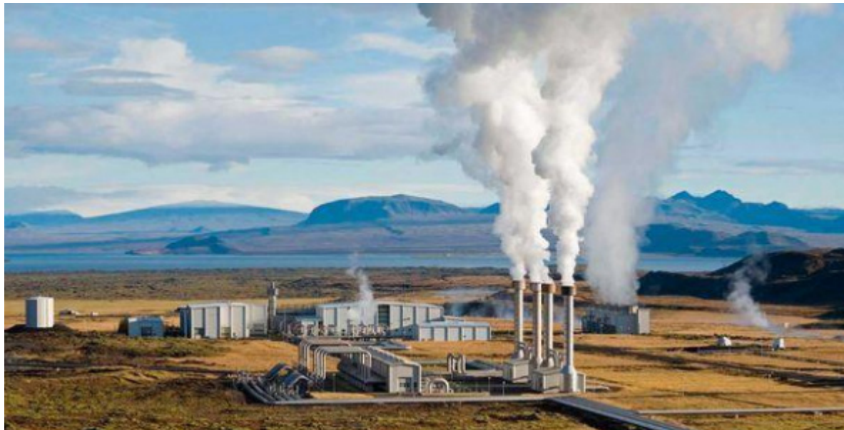
Kizildere III - Zorlu Geothermal Energy Power Plant
